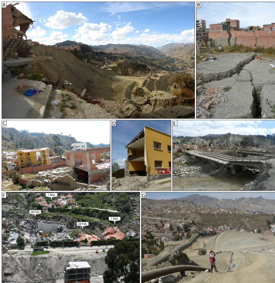
Figure 6. Impacts of the 2011 Pampahasi landslide. A. Headscarp (80 m height) along the east margin of Pampahasi Plateau (note excavator and trucks in lower middle ground for scale). B. Ground fissures in the northern part of the lower landslide mass. The wall in the background is ~2 m high. C. Back-tilted houses and apartment buildings on the northern part of the lower landslide mass (movement was from left to right). D. Community building with collapsed wall on the northern part of the lower landslide mass. E. Bridge across Río Irpavi that was deformed and shifted from its footings on 28 February near the centre of the landslide toe. F. Buildings on the southern part of the toe of the landslide that collapsed on 28 February and 1 March (dates of collapse shown; photo by M.A. Guzmán, 2 March 2011). G. Water service line ruptured by the landslide (upper pipe) and replacement water service line (lower pipe). See Figures 2B and 7C, D for locations of photographs. Photos taken by N.J. Roberts in May 2011 unless otherwise indicated.
