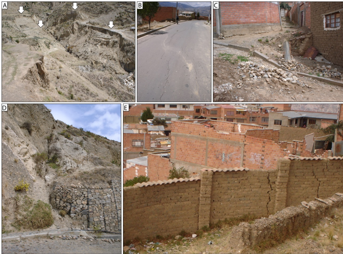
Figure 5. Field evidence of pre-failure creep in what would become the head region of the 2011 Pampahasi landslide. A. Small recent slumps (arrows) along Río Chujilluncani, ~400 m downslope from the east margin of Pampahasi Plateau. B. Minor cracking and centimeter-scale vertical offset of a paved road about 200 m east of, and 75 m below, the east margin of the plateau. C. Unpaved road with ~1 m displacement near the 2011 headscarp. D. Vertical offset along a gully ~75 m from the future south lateral margin of the 2011 landslide. The side of the gully nearer the middle of the 2011 landslide (right of the photo) has dropped ~0.5 m relative to the adjacent slope, causing deformation of the gabions and curb in the foreground. E. Cracks in an adobe wall (right foreground) and brick house (left middle ground) ~50 m downslope of the east margin of the plateau, corresponding to the middle of the 2011 landslide headscarp. See Figures 2A and 7A, B for locations of photographs. Photos taken by R.L. Hermanns in October 2005.
