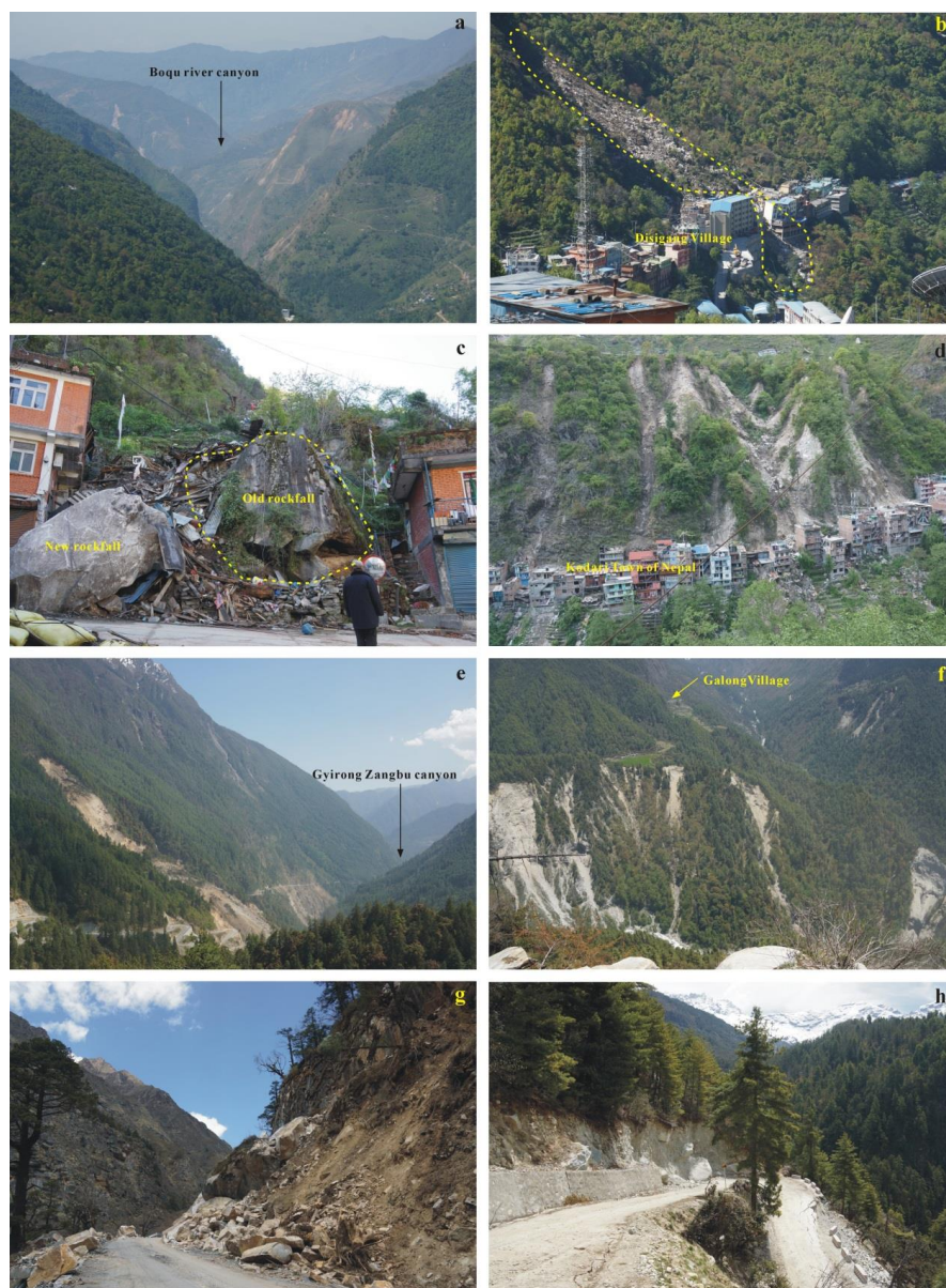
448 449 Fig. 5 Geologic effects caused during the Nepal earthquake: a, collapses in the Boqu valley; b, 450 collapse at Disigang Village (Site1, Fig. 4a); c. new and old rockfalls at Disigang Village (Site1, Fig. 451 4a); d, destroyed buildings in Kodari, Nepal (Site in Fig. 4a); e, large landslide in Chongse Village 452 (Site1, Fig. 4b); f, collapses in Galong Village(Site 7, Fig. 4b); g, collapses along highway from 453 Gyrong County to Jilong Town (Site 4, Fig. 4b); h, collapses and fissures along the highway from 454 Jilong to ChongseVillage (Site1, Fig. 4b). 455
