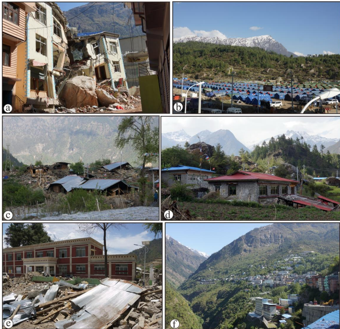
Fig. 4 Typical earthquake damage in southern Tibet and comparison of houses of different construction (locations shown in Fig. 5). Huge rockfall that smashed the resident committee office building at Disigang Village, about 0.7 km south of Zhangmu, where seven persons were killed (intensity IX) (site 1, Fig. 5a); b, A temporary settlement for earthquake survivors at Jilong; c, Destroyed houses of stone block masonry or adobe construction in Jifu Village southwest of Jilong (intensity VIII) (site 8, Fig. 5b); d, Houses of cement-bonded stone or brick construction in Jifu Village (intensity IX); e, Destroyed old houses and standing new buildings at Sale Town Primary School (intensity VIII) (site 7, Fig. 5b); f, Few collapsed houses at Zhangmu due to the brick structure or reinforced concrete construction (intensity IX).
