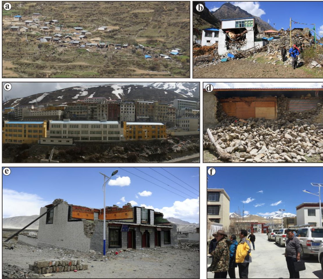
Fig. 3 The building damage resulting at different earthquake intensities: a, Many of the old stone pile or mud-brick houses collapsed, but the new brick houses rarely collapsed at Gangba Village in Sale Town in the intensity VIII zone; b, Similar building damage at Zhuobude Village of Rongxia Town in the intensity VIII zone; c, Most of buildings of brick-concrete structure did not collapse, but many walls showed obvious damage at Nyalam city located in the intensity VIII zone; d, Some walls of the stone-piled or mud-brick houses collapsed at Rema Village, Jilong County, in the intensity VII zone; e, Similar building damage at Chentang Town, Dinggyê county, in the intensity VII zone; f, Most of the houses remain intact and only few or individual walls of buildings had apparent small cracks at Jilong county city in the intensity VI zone.
