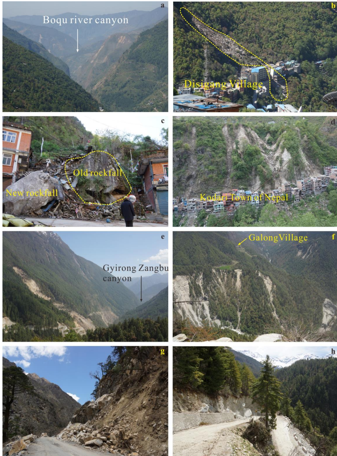
Fig. 6 Geologic effects caused during the Nepal earthquake: a, collapses in the Boqu valley; b, collapse at Disigang Village in the Boqu valley (Site1, Fig. 5a); c, new and old rockfalls at Disigang Village in the Boqu valley (Site1, Fig. 5a); d, destroyed buildings in Kodari, Nepal in the Boqu valley (Site in Fig. 4a); e, large landslide in Chongse Village in the Gyirong Zangbo valley (Site1, Fig. 5b); f, collapses in Galong Village in the Gyirong Zangbo valley (Site 7, Fig. 5b); g, collapses along highway from Gyirong County to Jilong Town in the Gyirong Zangbo
