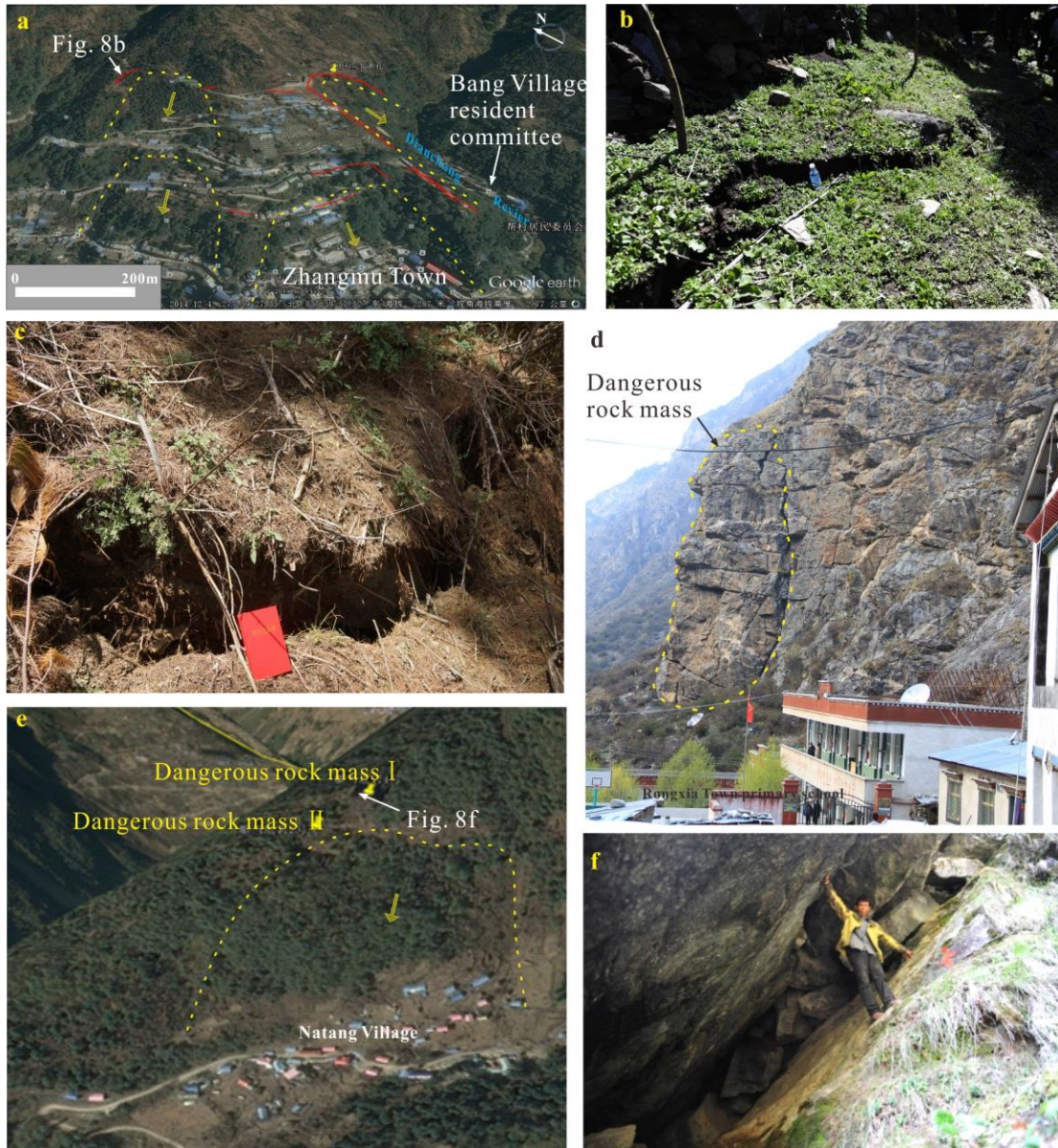
Fig. 8 Fissured and unstable rock masses formed by the earthquake that indicate hazards for additional landslides and rockfalls. Explanation: yellow dotted line, landslide group; arrow, slip direction; red line, new fissures formed during the Nepal earthquake; a, Old landslide group at Zhangmu. b. New fissure in the old landslide group at Zhangmu (site in Fig. 8a); c, Tension fissures at the back edge of Sale Village landslide (site7 in Fig. 5b); d, Dangerous rock mass at Rongxia Primary School (site 3 in Fig. 5c); e, Old landslide with unstable rock at Chentang Town (site 1 in Fig. 5d) and; f, Fissure between unstable rock and bedrock at Chentang (site in Fig. 8e).
