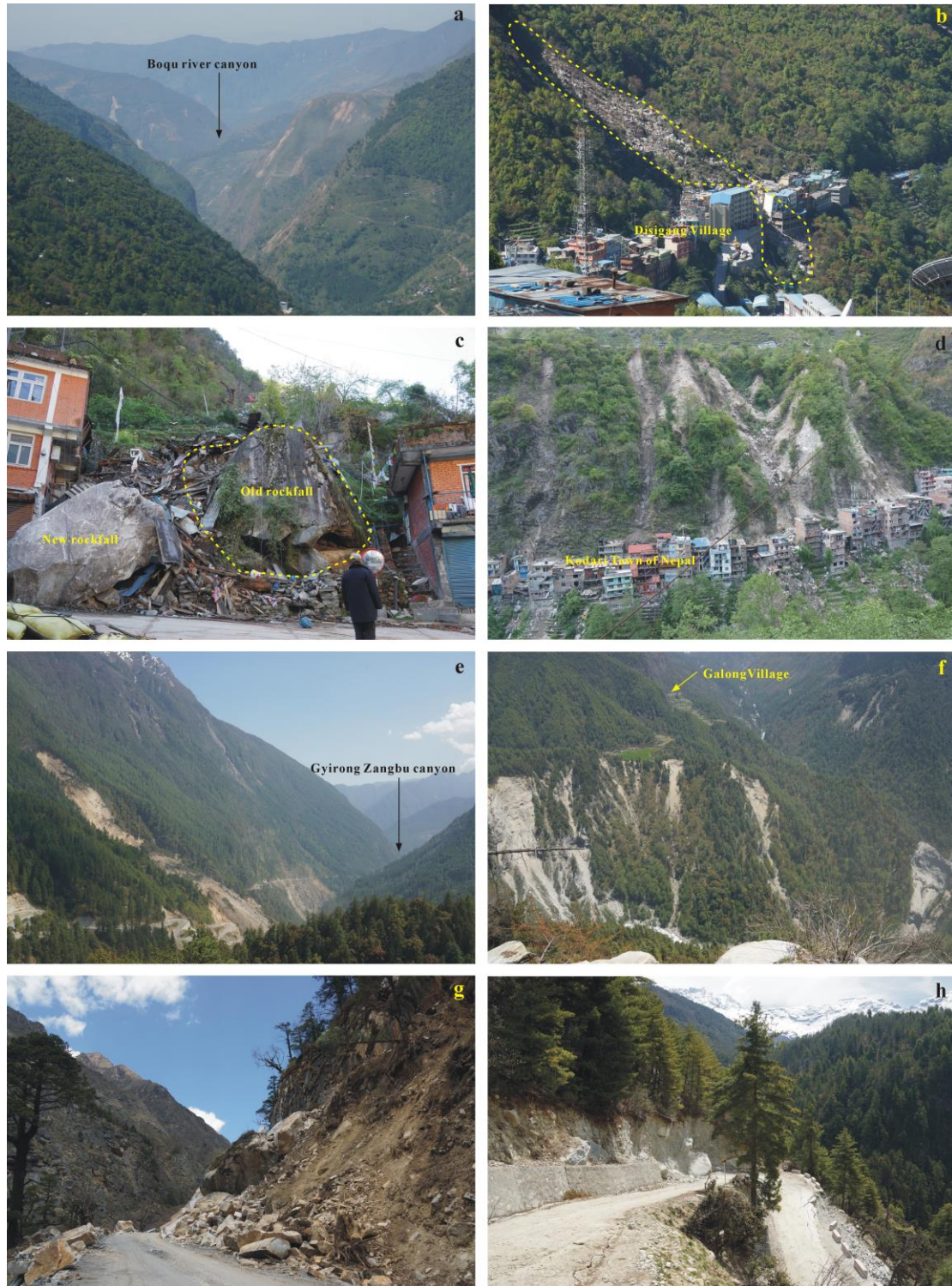
Fig. 6 Geologic effects caused during the Nepal earthquake: a, collapses in the Boqu valley; b, collapse at Disigang Village in the Boqu valley (Site1, Fig. 5a); c, new and old rockfalls at Disigang Village in the Boqu valley (Site1, Fig. 5a); d, destroyed buildings in Kodari, Nepal in the Boqu valley (Site in Fig. 4a); e, large landslide in Chongse Village in the Gyirong Zangbu valley (Site1, Fig. 5b); f, collapses in Galong Village in the Gyirong Zangbu valley (Site 7, Fig. 5b); g, collapses along highway from Gyirong County to Jilong Town in the Gyirong Zangbu
