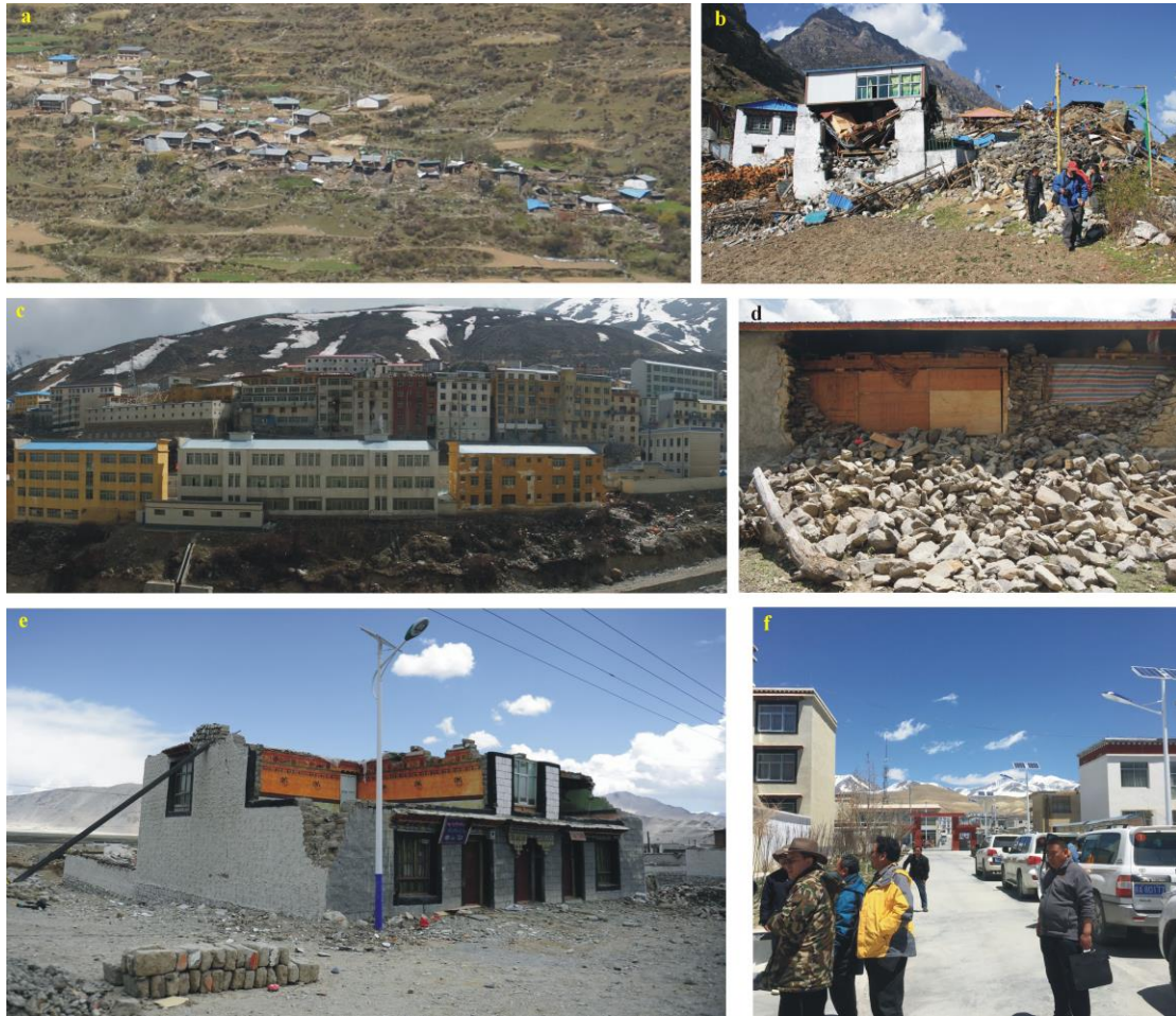
Fig. 3 The building damage resulting at different earthquake intensities: a, Many of the old stone pile or mud-brick houses collapsed, but the new brick houses rarely collapsed at Gangba Village in Sale Town in the intensity VIII zone; b, Similar building damage at Zhuobude Village of Rongxia Town in the intensity VIII zone; c, Most of buildings of brick-concrete structure did not collapse, but many walls showed obvious damage at Nyalam city located in the intensity VIII zone; d, Some walls of the stone-piled or mud-brick houses collapsed at Rema Village, Jilong County, in the intensity VII zone; e, Similar building damage at Chentang Town, Dinggyê county, in the intensity VII zone; f, Most of the houses remain intact and only few or individual walls of buildings had apparent small cracks at Jilong county city in the intensity VI zone.
