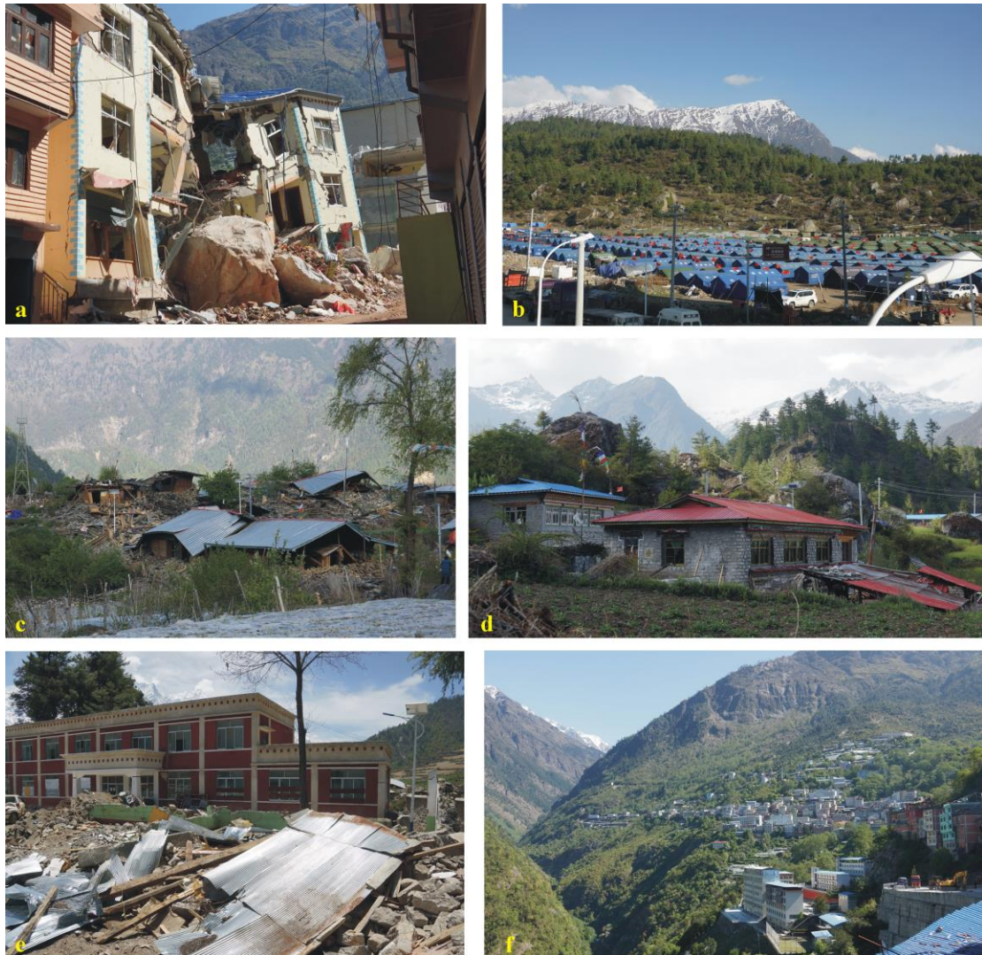
Fig. 4 Typical earthquake damage in southern Tibet and comparison of houses of different construction (locations shown in Fig. 5). Huge rockfall that smashed the resident committee office building at Disigang Village, about 0.7 km south of Zhangmu, where seven persons were killed (intensity IX) (site 1, Fig. 5a); b, A temporary settlement for earthquake survivors at Jilong; c, Destroyed houses of stone block masonry or adobe construction in Jifu Village southwest of Jilong (intensity VIII) (site 8, Fig. 5b); d, Houses of cement-bonded stone or brick construction in Jifu Village (intensity IX); e, Destroyed old houses and standing new buildings at Sale Town Primary School (intensity VIII) (site 7, Fig. 5b); f, Few collapsed houses at Zhangmu due to the brick structure or reinforced concrete construction (intensity IX).
