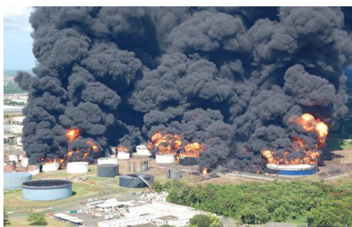
Figure 10. Fire domino effect in a tank farm in Puerto Rico in 2009 (CSB, 2015).
