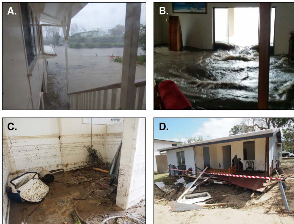
Figure 10: Flooding (A), water ingress (B), interior (C) and exterior (D) damage to property at Wilson Beach. (C) and (D) are authors' own images; (A) and (B) were taken by residents at Wilson Beach, reproduced with their permission for this paper.
