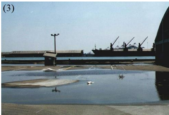
Figure 6. Photos showing liquefaction-induced hazards during the Chi-Chi earthquake and the 2011 Tohoku earthquake: (1) Sand boils in Chikusei city; (2) Ground cracks at Arakawa River in Toda city; (3) Settlement at Taichung Port ( http://www.ces.clemson.edu/chichi/TW-LIQ/Liq-Album/Settlement-7.htm ); (4) Lateral spread induced failure of a dike in Nantou ( http://www.ces.clemson.edu/chichi/TW-LIQ/Liq-Album/LatSpread-3.htm ).
