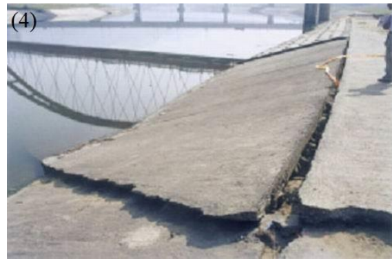
Figure 6. Photos showing liquefaction-induced hazards during the Chi-Chi earthquake and the 2011 Tohoku earthquake: (1) Sand boils in Chikusei city; (2) Ground cracks at Arakawa River in Toda city; (3) Settlement at Taichung Port ( http://www.ces.clemson.edu/chichi/TW-LIQ/Liq-Album/Settlement-7.htm ); (4) Lateral spread induced failure of a dike in Nantou ( http://www.ces.clemson.edu/chichi/TW-LIQ/Liq-Album/LatSpread-3.htm ).
