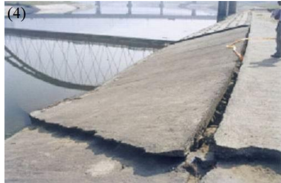
Figure 6. Photos showing liquefaction-induced hazards during the Chi-Chi earthquake and the 2011 Tohoku earthquake: (1) Sand boils in Chikusei city; (2) Ground cracks at Arakawa River in Toda city; (3) Settlement at Taichung Port ( http://www.ces.clemson.edu/chichi/TW-LIQ/Liq-Album/Settlement-7.htm ); (4) Lateral spread induced failure of a dike in Nantou ( http://www.ces.clemson.edu/chichi/TW-LIQ/Liq-Album/LatSpread-3.htm ).
