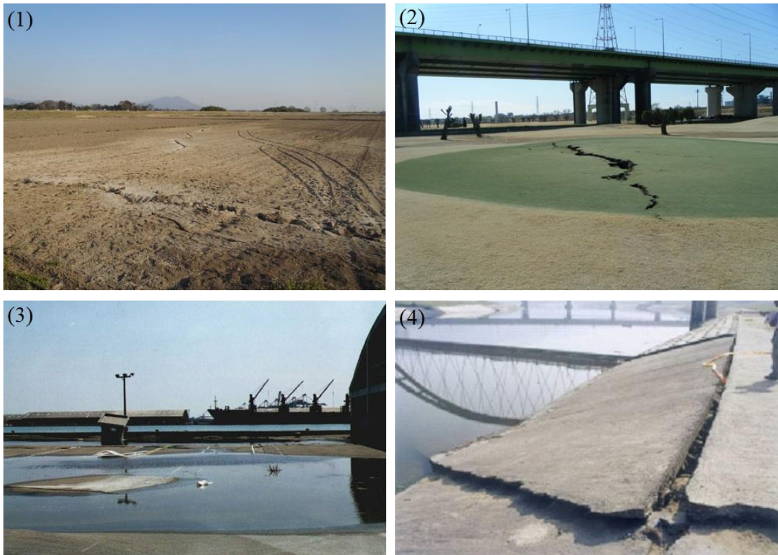
Figure 6. Photos showing liquefaction-induced hazards during the Chi-Chi earthquake and the 2011 Tohoku earthquake: (1) Sand boils in Chikusei city; (2) Ground cracks at Arakawa River in Toda city; (3) Settlement at Taichung Port ( http://www.ces.clemson.edu/chichi/TW-LIQ/Liq-Album/Settlement-7.htm ); (4) Lateral spread induced failure of a dike in Nantou ( http://www.ces.clemson.edu/chichi/TW-
