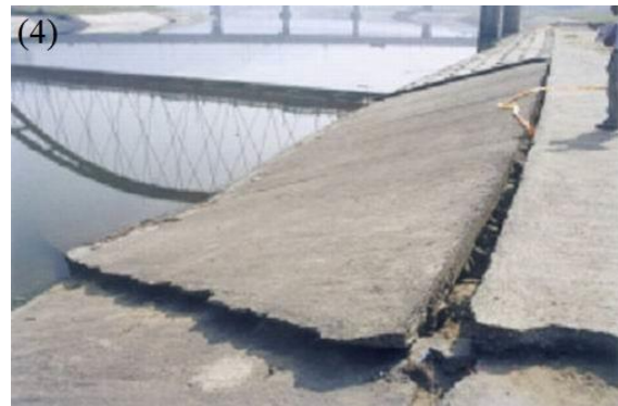
Figure 5. Photos showing liquefaction-induced hazards during the Chi-Chi earthquake and the 2011 Tohoku earthquake: (1) Sand boils in Chikusei city; (2) Ground cracks at Arakawa River in Toda city; (3) Settlement at Taichung Port ( http://www.ces.clemson.edu/chichi/TW-LIQ/Liq-Album/Settlement-7.htm ); (4) Lateral spread induced failure of a dike in Nantou ( http://www.ces.clemson.edu/chichi/TW-LIQ/Liq-Album/LatSpread-3.htm ).
