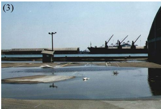
Figure 5. Photos showing liquefaction-induced hazards during the Chi-Chi earthquake and the 2011 Tohoku earthquake: (1) Sand boils in Chikusei city; (2) Ground cracks at Arakawa River in Toda city; (3) Settlement at Taichung Port ( http://www.ces.clemson.edu/chichi/TW-LIQ/Liq-Album/Settlement-7.htm ); (4) Lateral spread induced failure of a dike in Nantou ( http://www.ces.clemson.edu/chichi/TW-LIQ/Liq-Album/LatSpread-3.htm ).
