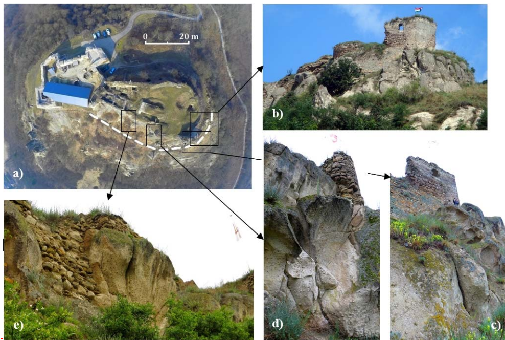
Figure.4. Studied southern cliff faces (clockwise): a) image of the castle obtained by RPAS with marked details; b) distant view of the eastern part of the cliff section; c) weathered rounded cliff with larger taffoni; d) vertical to sub-vertical cliff face with steep joints and traces of rock fall; e) steep cliffs dissected by joints.
