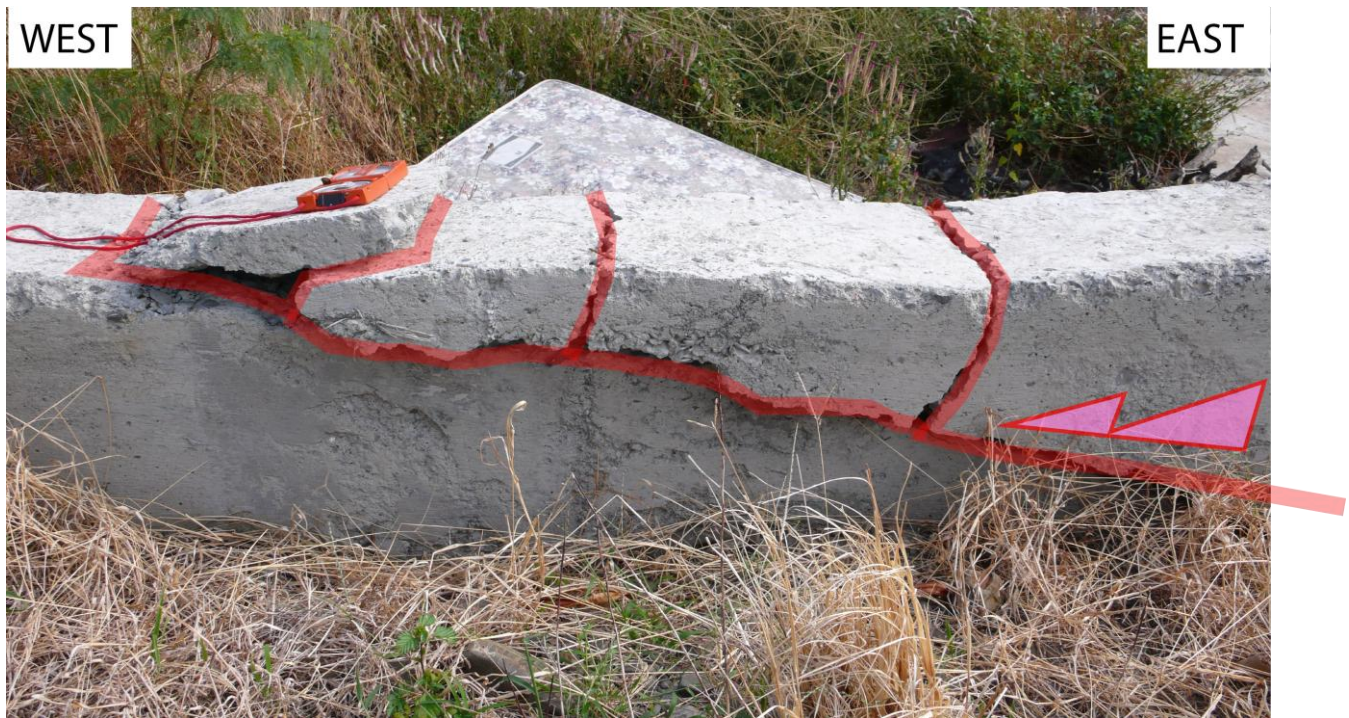
Figure 6: Field work photograph of compressive features affecting recent concrete dykes after the Hengchun earthquake (Dec. 26 th 2006, M_L=7.0 ), see location on Fig. 1 near the Fang-Shan village (22.26°N, 120.66°E). The red compass gives the scale of the outcropping deformation (20cm). Thrust associated with three back-thrusts highlighting a small pop-up (below the compass). The red arrow reveals the thrusting component that affects the new concrete dykes.
