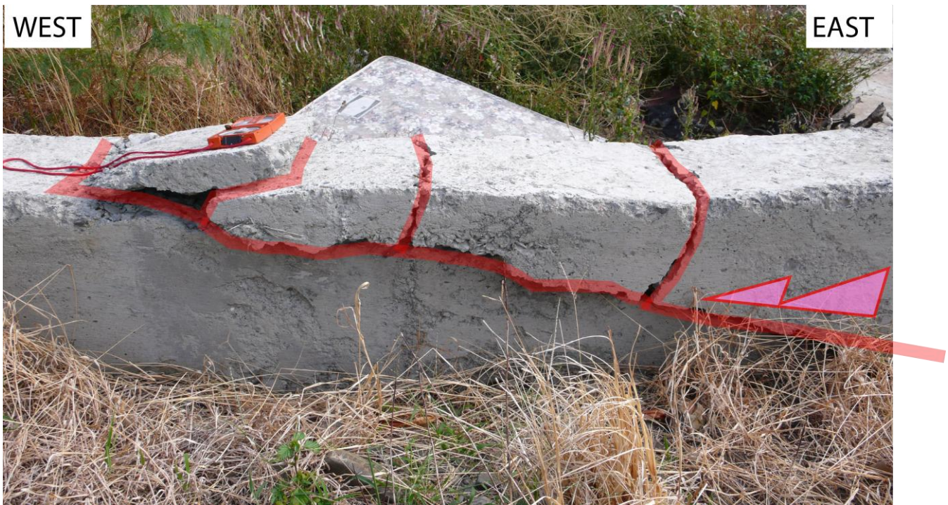
5 Figure 6: Field work photograph of compressive features affecting recent concrete dykes after the Hengchun earthquake (Dec. 26 th 2006, M_L=7.0 ), see location on Fig. 1 near the Fang-Shan village (22.26°N, 120.66°E). The red compass gives the scale of the outcropping deformation (20cm). Thrust associated with three back-thrusts highlighting a small pop-up (below the compass). The red arrow reveals the thrusting component that affects the new concrete dykes.
