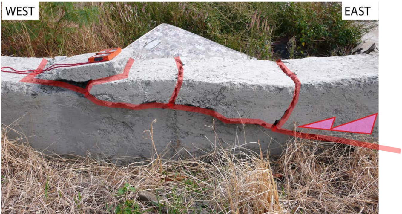
5 Figure 5: Field work photograph of compressive features affecting recent concrete dykes after the Hengchun earthquake (Dec. 26 th 2006, M_L=7.0 ), see location on Fig. 1 near the Fang-Shan village (22.26°N, 120.66°E). The red compass gives the scale of the outcropping deformation (20cm). Thrust associated with three back-thrusts highlighting a small pop-up (below the compass). The red arrow reveals the thrusting component that affects the new concrete dykes
