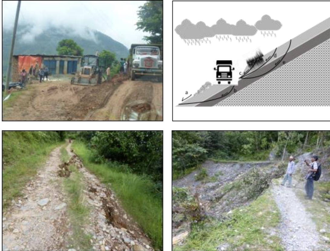
Figure 1. Informal, rural roads in Sindhupalchok District, Nepal. (Top left) Earth-moving equipment is hired by villagers to expand footpaths into roads that bring goods and services to isolated locations. (Top right) There are 5 primary modes of potentially damaging mass movements caused by informal road construction- a) debris flows from excavated material stored on the downslope side of the road; b) Deeper seated landslides that are accommodated by poor road drainage; c) Shallow failures close to the road caused by oversteepened road cuts that can be mitigated by planting; d) Shallow landslides caused by oversteepening that include potentially stabilising roots from vegetation; e) Deeper seated failures below root zone related to road cuts. (Bottom left and right) Without proper engineering (slope gradients, drainage, etc.), landslides are triggered on these rural roads during heavy monsoonal rains, damaging land, structures, and roads, and endangering human lives and livelihoods.
