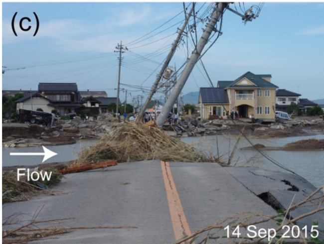
Figure 9: Photos of the study area. (a) Crevasse channel (breach scouring) near the levee. Note the building still standing after the flood in the center of the photo. (b) Sand splay in the southern part of the study area. (c) Damaged prefectural road beside the breached levee. (d) Overturned and transported house. Note the sandy mound in the downstream direction from the house. See
