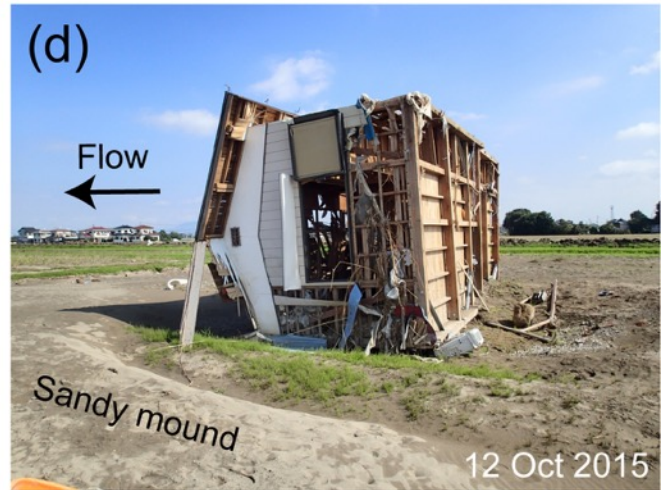
Figure 9: Photos of the study area. (a) Crevasse channel (breach scouring) near the levee. Note the building still standing after the flood in the center of the photo. (b) Sand splay in the southern part of the study area. (c) Damaged prefectural road beside the breached levee. (d) Overturned and transported house. Note the sandy mound in the downstream direction from the house. See
