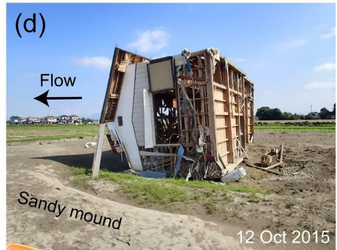
Figure 9: Photos of the study area. (a) Crevasse channel (breach scouring) near the levee. Note the building still standing after the flood in the center of the photos. (b) Sand splay in the southern part of the study area. (c) Damaged prefectural road beside the breached levee. (d) Overturned and transported house. Note a sandy mound in the downstream direction from the house. See Fig. 5 3c for the photo locations. Photos were taken by A. Izumida and T. Sugai.
