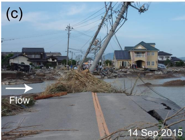
Figure 9: Photos of the study area. (a) Crevasse channel (breach scouring) near the levee. Note the building still standing after the flood in the center of the photos. (b) Sand splay in the southern part of the study area. (c) Damaged prefectural road beside the breached levee. (d) Overturned and transported house. Note a sandy mound in the downstream direction from the house. See Fig. 5 3c for the photo locations. Photos were taken by A. Izumida and T. Sugai.
