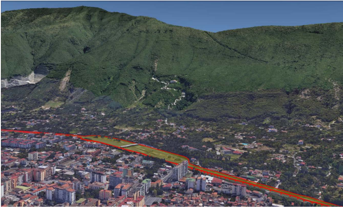
Figure 3. Infrastructure-scale view of the study area with the A3 Salerno-Reggio Calabria motorway (boundaries marked in red)
