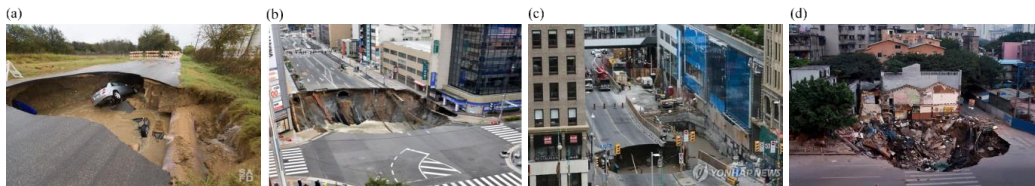
91 Figure 3. Ground subsidence nearby subway of urban railway in the US, Canada, Japan, and China. Texas in the US (a). 92 Fukuoka in Japan (b). Ottawa in Canada (c). Guangzhou in China (d).
