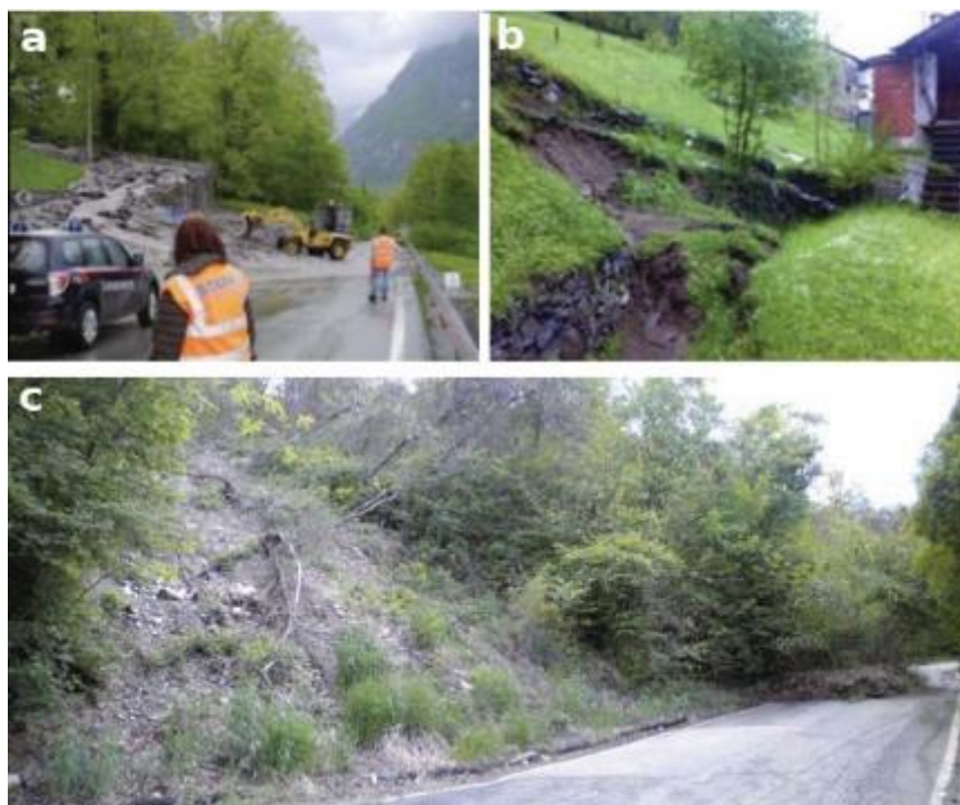
Fig. 14: Some examples of slope phenomena recorded during rainfall event. a) Road interrupted by a debris flow; b) a building hit by small rotational slide; c) shallow landslides on a road (source: Regione Piemonte).
