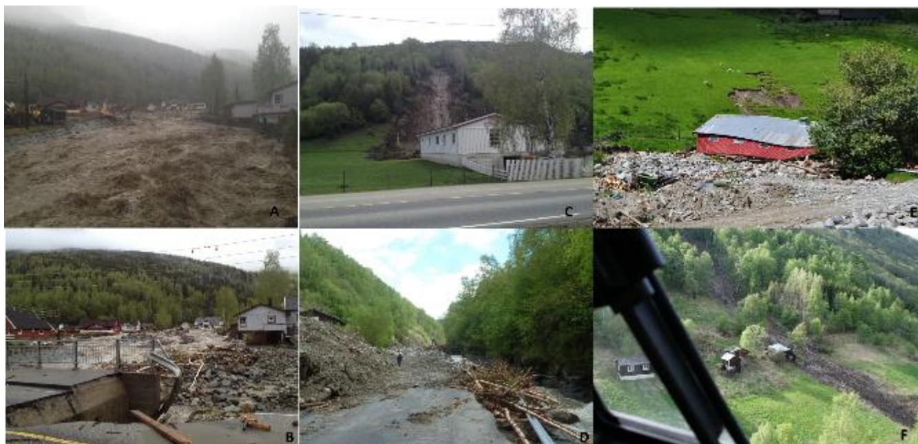
Fig. 16: Flood and landslides at Kvam, Nord Frøn, Oppland county 22 nd May 2013. A) and B) Flood and flood damages at 5 Kvam; C) Debris slide at Ringebu; D) debris flow at Veikleåadalen E) shallow debris slide and debris flow deposits at Kvam; F) Debris flow at Veikleåadalen (Source: NVE).
