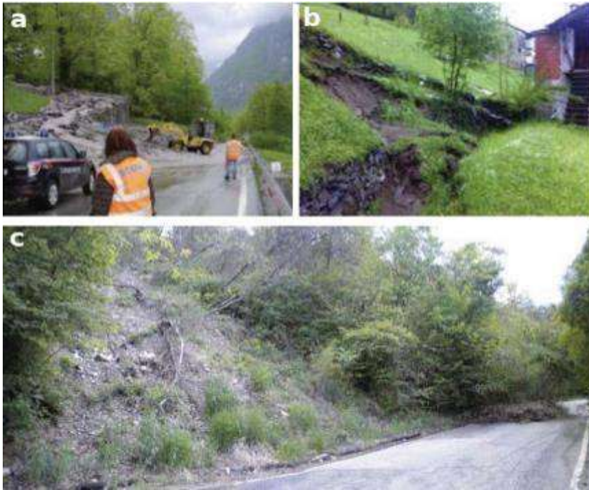
Fig. 15: Some examples of slope phenomena recorded during rainfall event. a) Road interrupted by a debris flow; b) a building hit by small rotational slide; c) shallow landslides on a road (source: Regione Piemonte).
