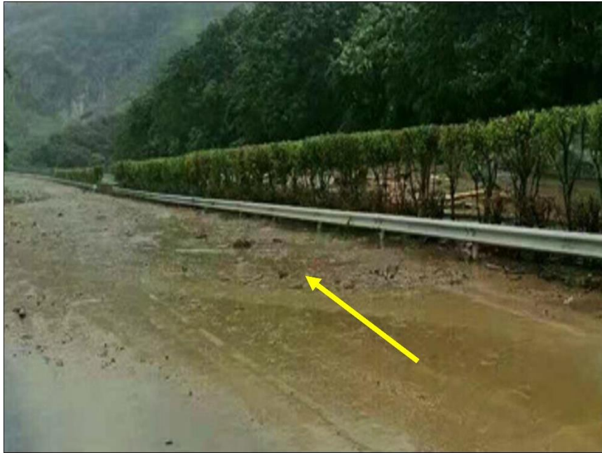
Figure 1. Soil erosion produced by rainwash on a slope after rainfall
