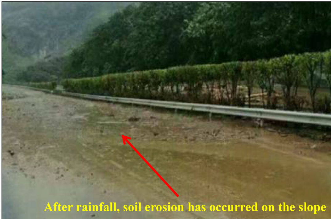
Fig. 2. Soil erosion produced by rainwash on slope
