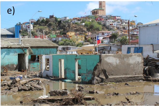
Figure 2: Photographs of structures undamaged and masonry houses damaged by the September 16 th 2015 tsunami in the Coquimbo area. The red letter d indicates the observed tsunami inundation depth. All photos were taken on September 22 nd of 2015.
