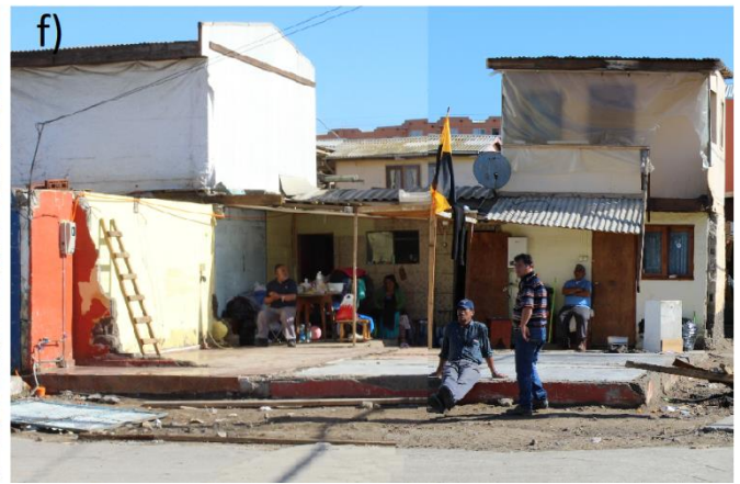
Figure 2: Photographs of surveyed masonry houses after the September 16 th 2015 tsunami in the Coquimbo area. The red letter d indicates the observed tsunami inundation depth. All photos were taken on September 22 nd of 2015. a) and b) Houses with no damage. c) 2-story house with moderate damage. d) 1-story house with major damage. e) 1-story house with complete damage. f) Washed away structure.
