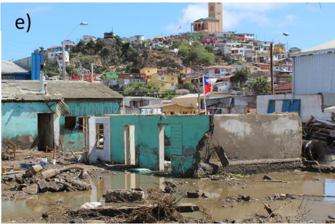
Figure 2: Photographs of surveyed masonry houses after the September 16 th 2015 tsunami in the Coquimbo area. The red letter d indicates the observed tsunami inundation depth. All photos were taken on September 22 nd of 2015. a) and b) Houses with no damage. c) 2-story house with moderate damage. d) 1-story house with major damage. e) 1-story house with complete damage. f) Washed away structure.
