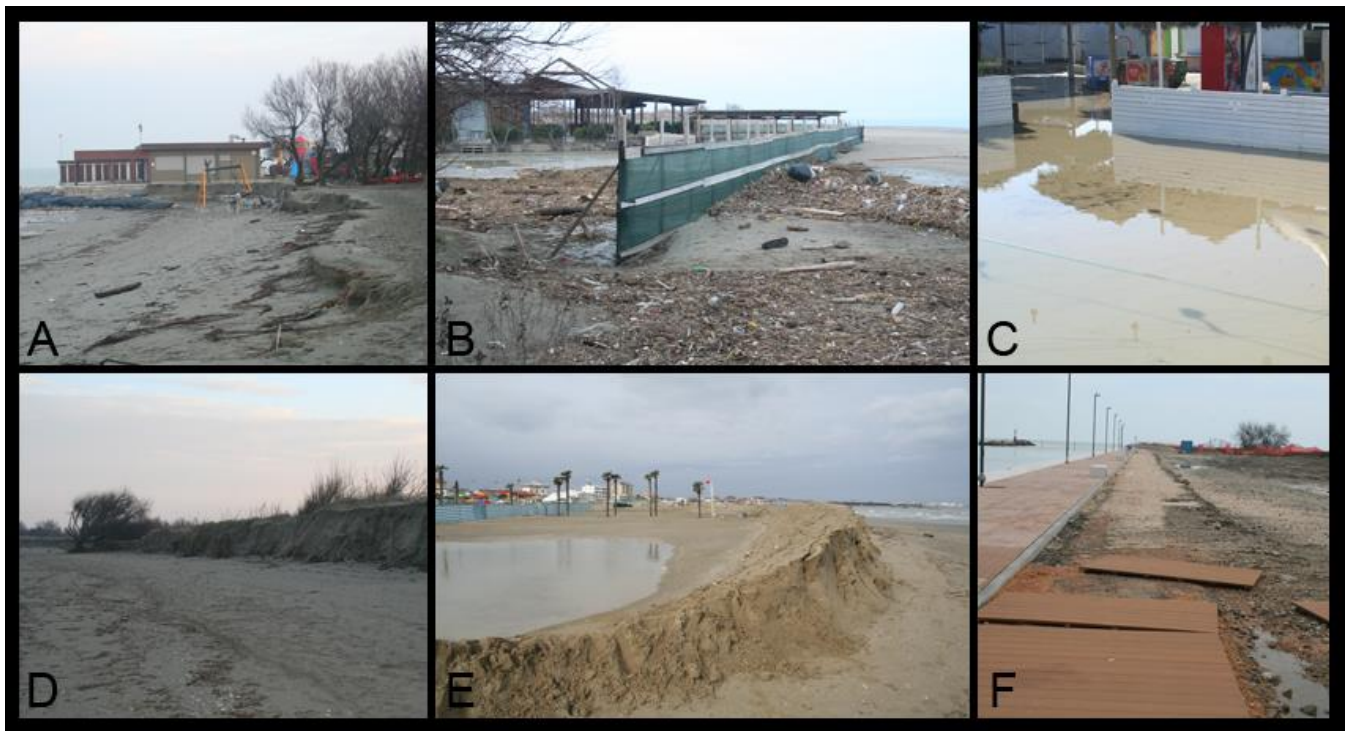
Figure 3: Impacts of the event in February 2015 on the Lido degli Estensi-Spina case study area. Impacts of erosion and flooding on concessions at Lido di Spina south (A, B) and Lido degli Estensi (C); sandy scarp due to the erosion of the dune in the south of Lido di Spina (D); eroded Winter Dune in Porto Garibaldi (E); damages to the Porto Canale front at the Lido degli Estensi (F).
