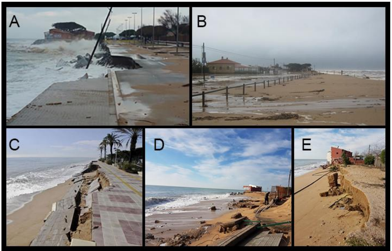
Figure 2: Impacts on the Tordera Delta. Destruction of a road at Malgrat (A); overwash at campsites north of the river mouth (B); destruction of the promenade north of the river mouth (C); beach erosion, and damage to utilities and buildings at Malgrat (D and E).
