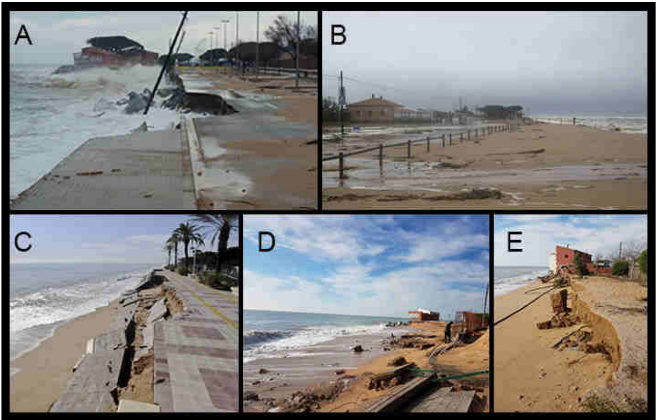
Figure 2: Impacts on the Tordera Delta. Destruction of a road at Malgrat (A); overwash at campsites north of the river mouth (B); destruction of the promenade north of the river mouth (C); beach erosion, and damage to utilities and buildings at Malgrat (D and E).
