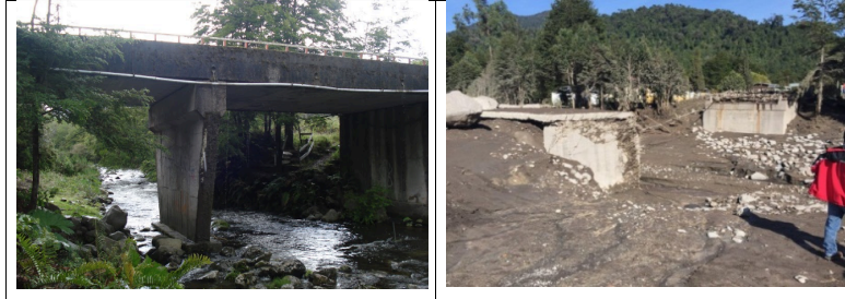
Figure 2: (a) Original Rio Blanco Bridge (Chile) (MOP, 2015). (b) Rio Blanco Bridge (Chile) after lahar flow of the Calbuco volcano eruption in 2015 (MOP, 2015).
