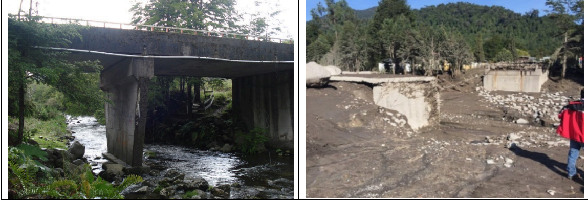
Figure 2: (a) Original Río Blanco Bridge (Chile) (MOP, 2015). (b) Río Blanco Bridge (Chile) after lahar flow of the Calbuco volcano eruption in 2015 (MOP, 2015).
