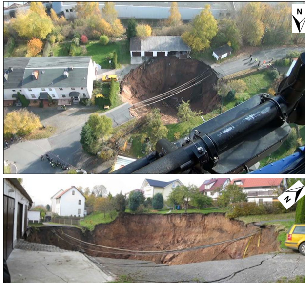
Figure 2. Photographs showing the sinkhole in Schmalkalden that opened up on 1st November 2010. It is 26 to 30 m in diameter and 12 to 17 m in depth (TLUG, 2010).
