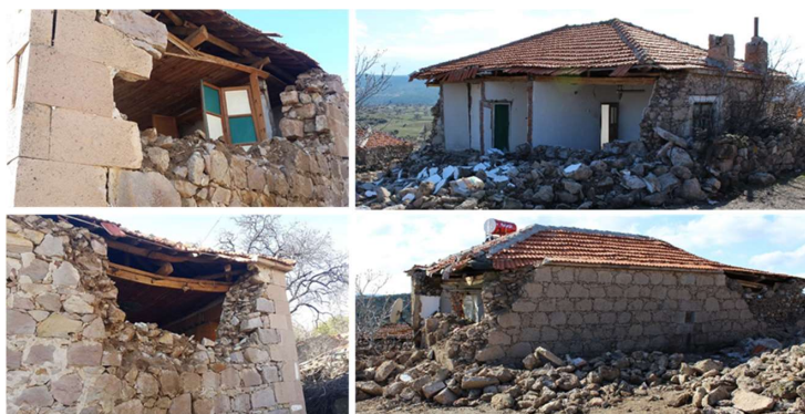
Figure 17 Out of plane failures depending on improper wall thickness and/or height-length ratio
