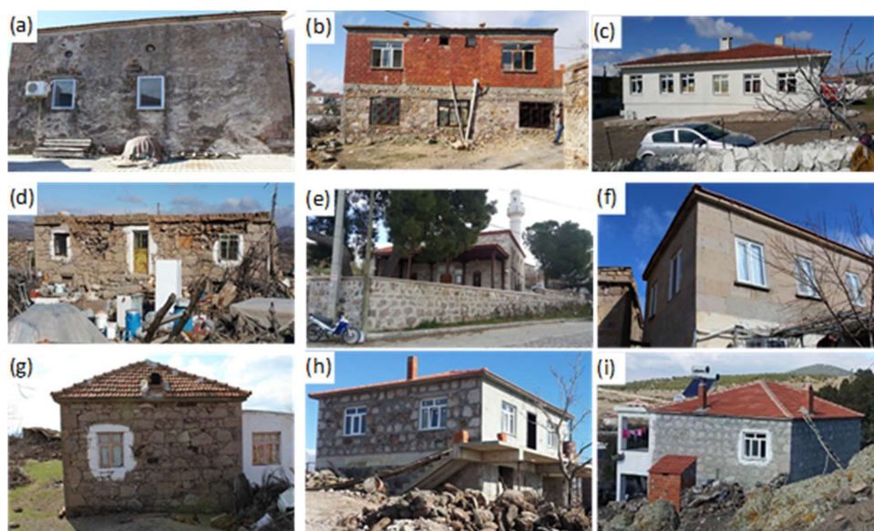
15 Figure 5 Existing building types in reconnaissance area: a) hatıl dwelling b) stone and brick in cement mortar, c) engineered RC building d) hatıl building with heavy roof, e) historical masonry with cut stone, f) cut stone without mortar, g) stone without mortar, h), i) stone in cement mortar with reinforced concrete.
