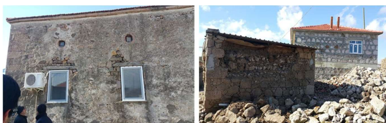
Figure 15 Examples of undamaged dwellings
