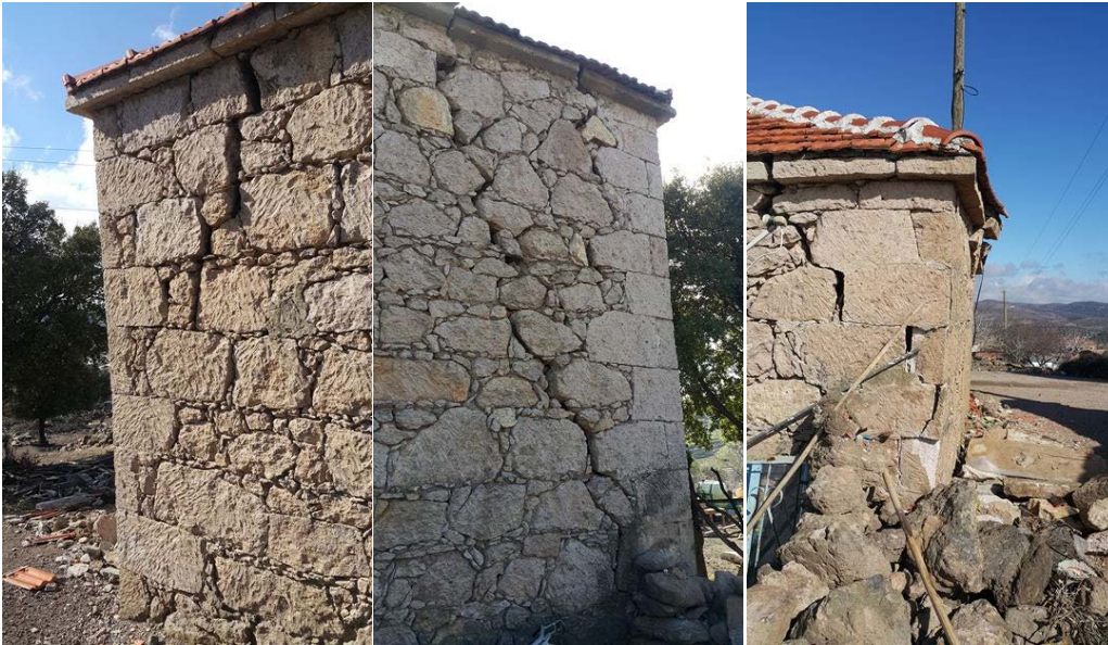
Figure 23: Examples of diagonal shear cracking
