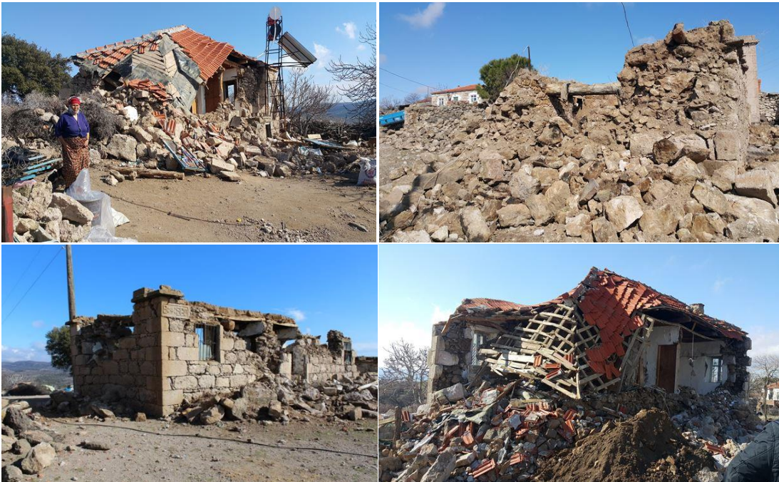
Figure 16: Examples of totally collapsed structures from Ayvacık, Çanakkale 2017 earthquake swarm
