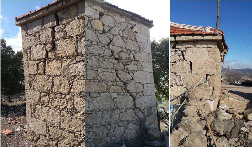
Figure 23: Examples of diagonal shear cracking
