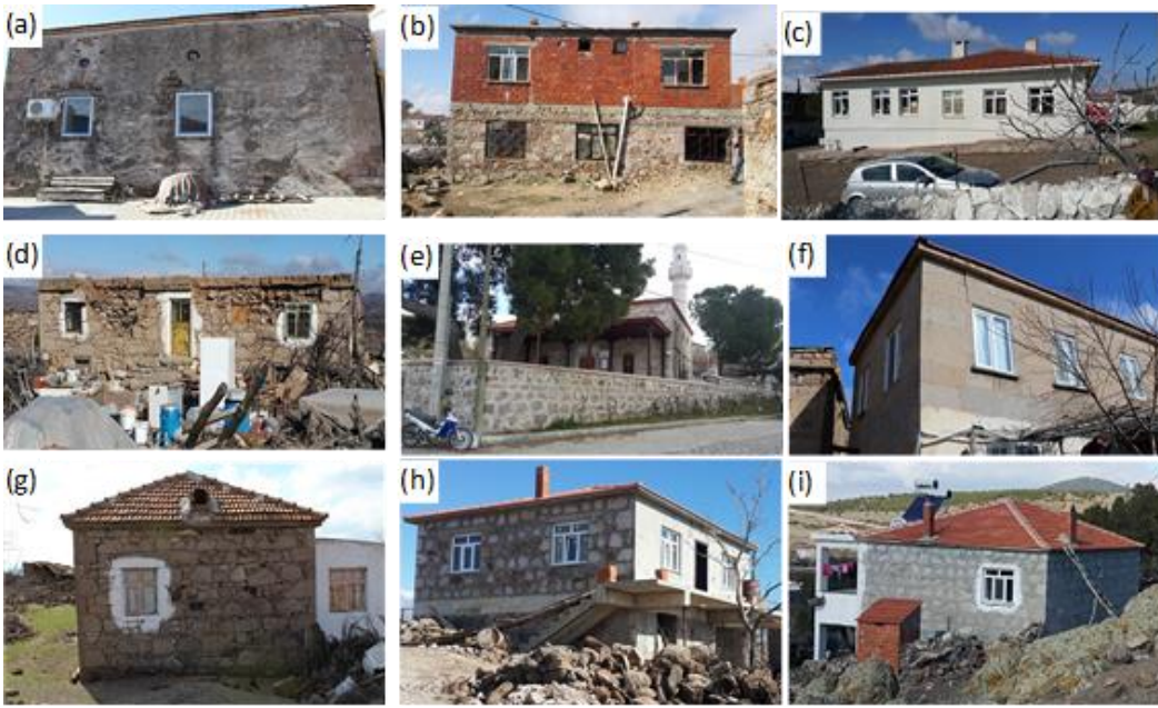
Figure 4: Existing building types in reconnaissance area: a) hatıl dwelling b) stone and brick in cement mortar, c) engineered RC building d) hatıl building with heavy roof, e) historical masonry with cut stone, f) cut stone without mortar, g) stone without mortar, h), i) stone in cement mortar with reinforced concrete.
