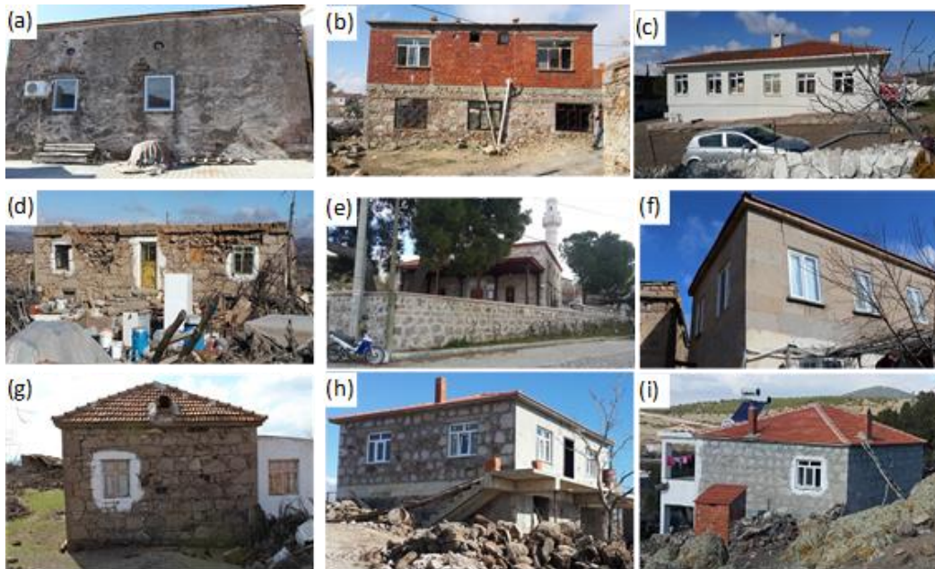
5 Figure 4: Existing building types in reconnaissance area: a) hatıl dwelling b) stone and brick in cement mortar, c) engineered RC building d) hatıl building with heavy roof, e) historical masonry with cut stone, f) cut stone without mortar, g) stone without mortar, h), i) stone in cement mortar with reinforced concrete.
