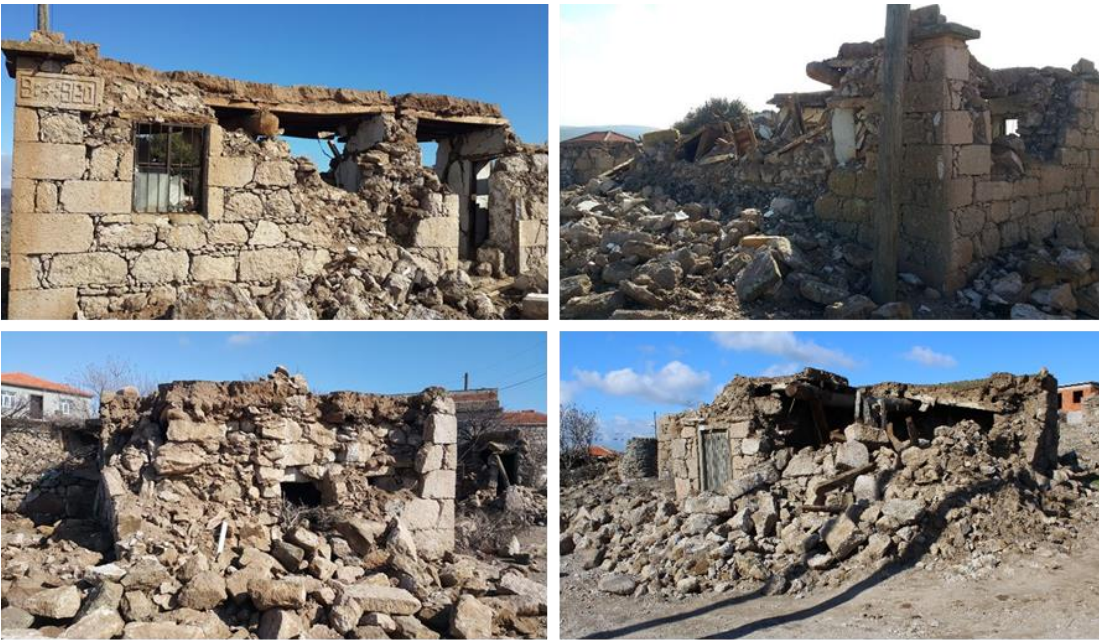
Figure 21: Examples of heavy earth wall collapse
