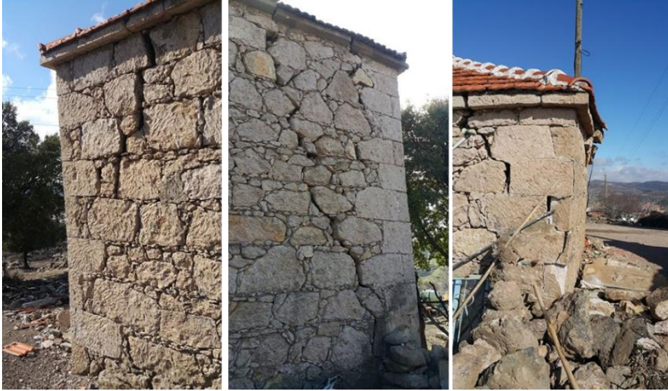
Figure 23: Examples of diagonal shear cracking
