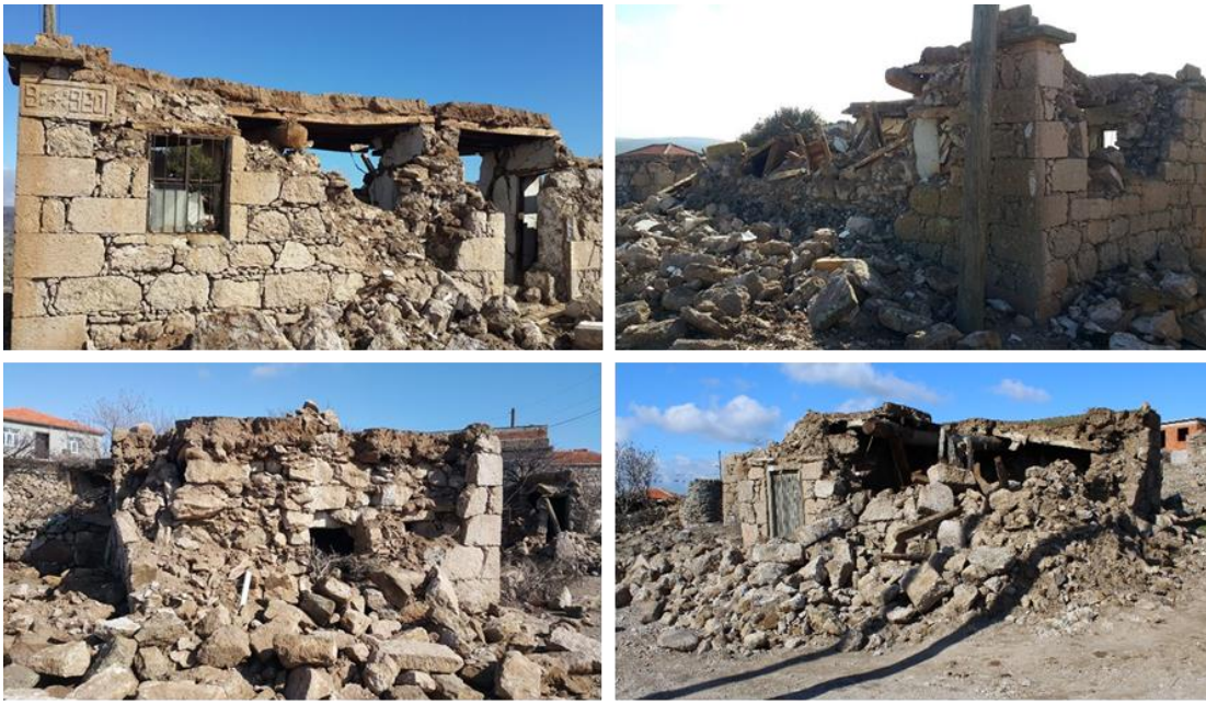
Figure 21: Examples of heavy earth wall collapse
