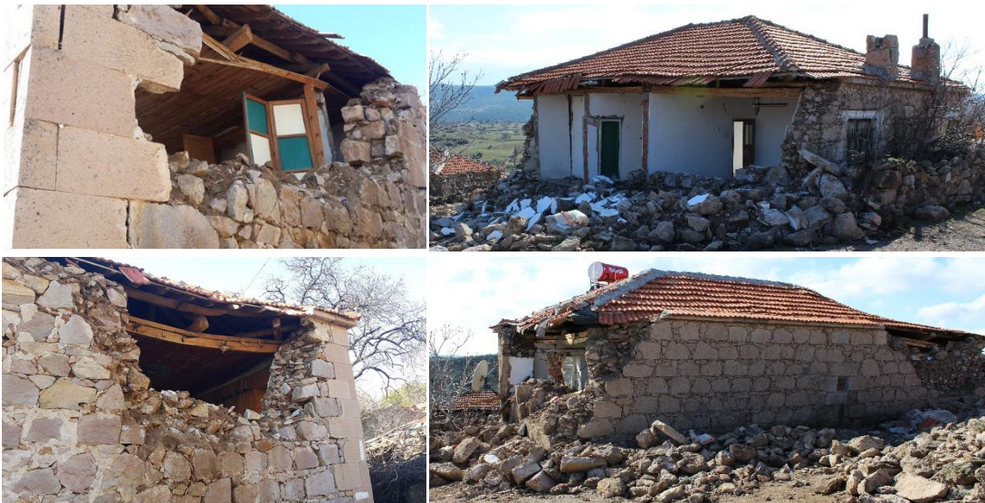
Figure 24: Out of plane failures due to improper wall thickness and/or height-length ratio
