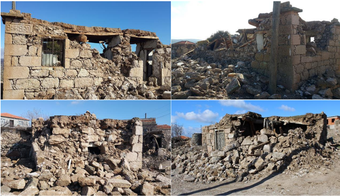
Figure 21: Examples of heavy earth wall collapse
