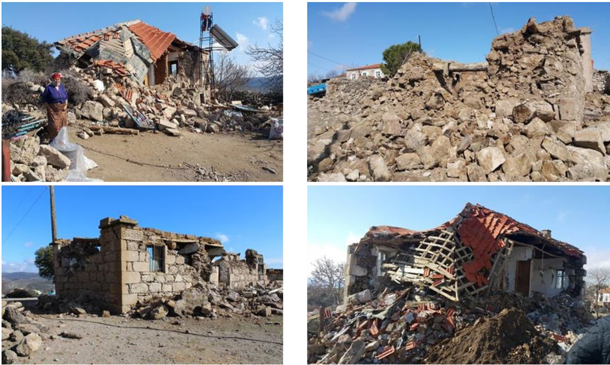
Figure 16:5 Examples of Totally totally collapsed examples-structures from Ayvacık, Çanakkale 2017 earthquakes swarm
