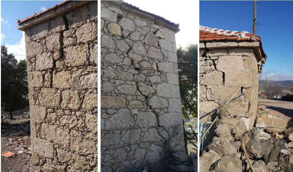
Figure 223: Examples of diagonal shear cracking
