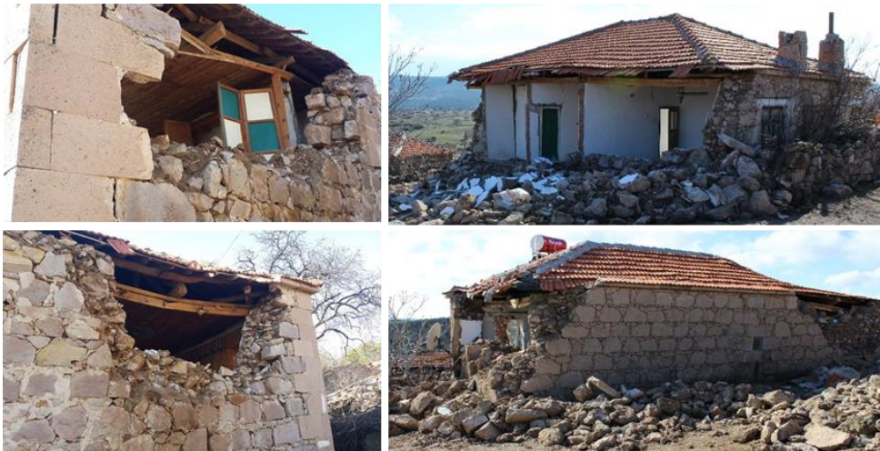
Figure 243: Out of plane failures depending on due to improper wall thickness and/or height-length ratio
