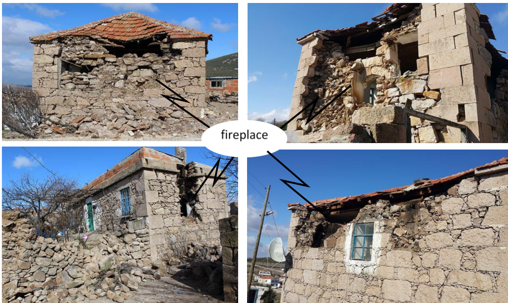
Figure 201920.: Examples of out of plane collapse due to wall cavity
