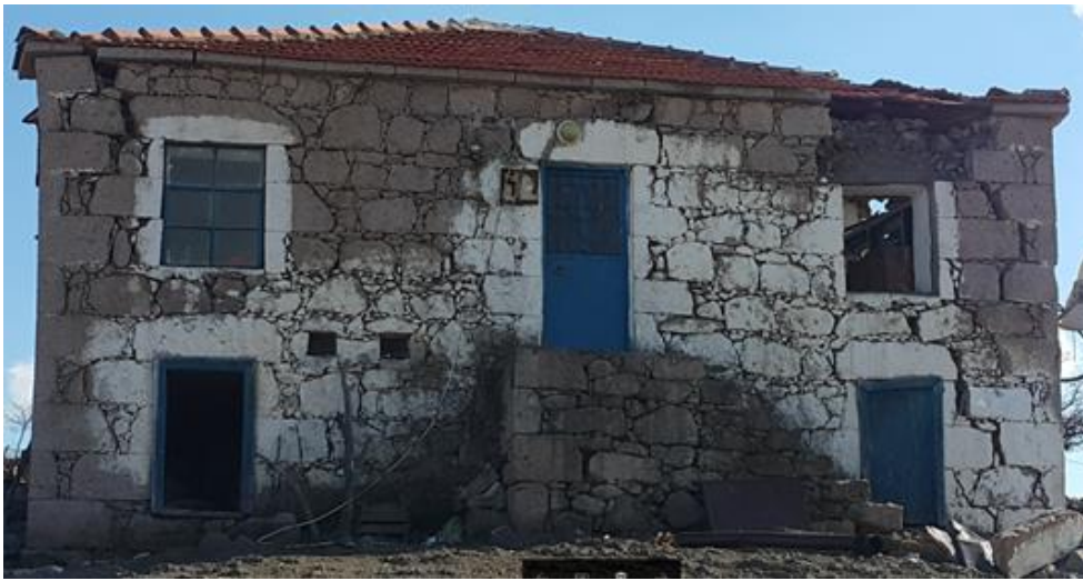
Figure 17617: An example of a damaged dwelling due to inadequate interlocking
