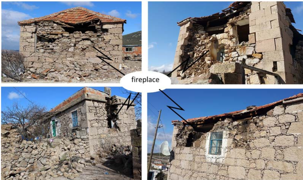
Figure 19 Examples of out of plane collapse due to wall cavity
