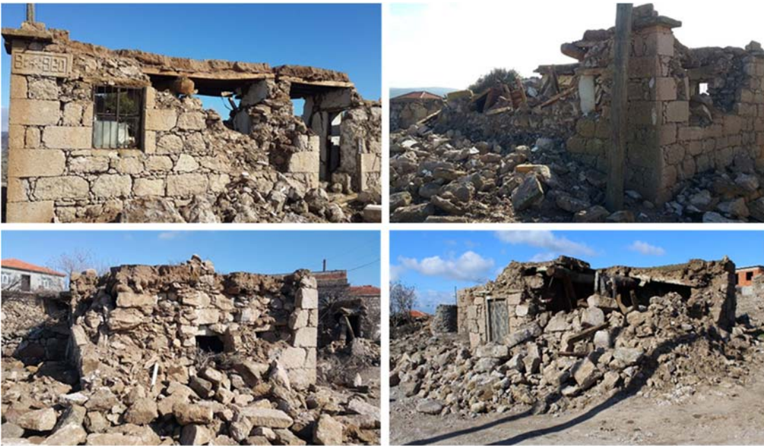
Figure 20 Examples of heavy earth wall collapse
