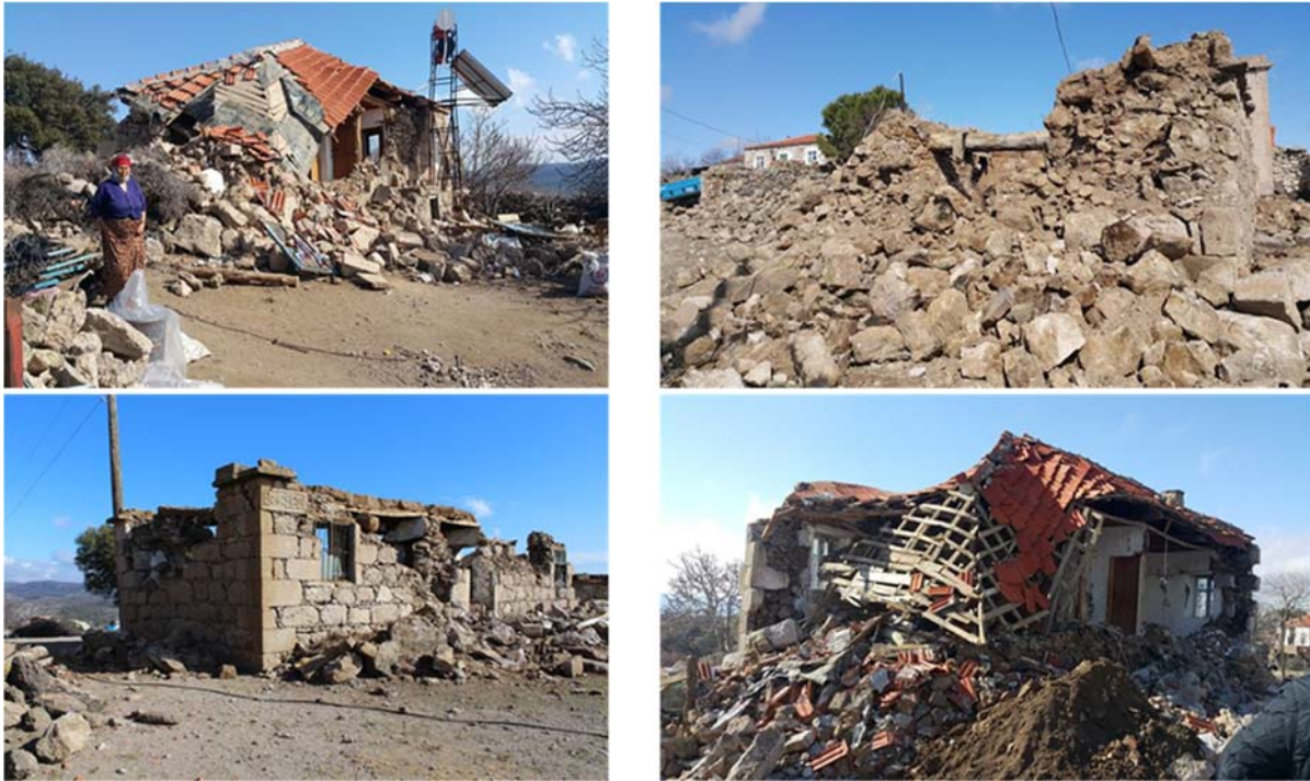
5 Figure 15 Totally collapsed examples from Ayvacık, Çanakkale 2017 earthquakes swarm
