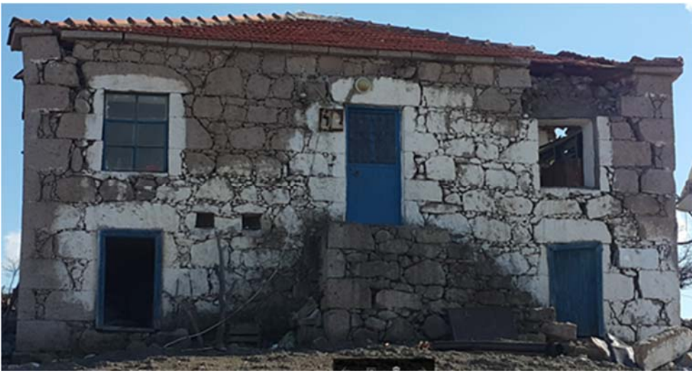
Figure 16 An example of damaged dwelling due to inadequate interlocking
