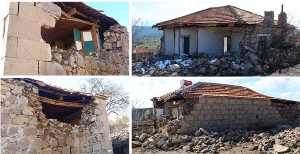
10 Figure 23 Out of plane failures depending on improper wall thickness and/or height-length ratio
