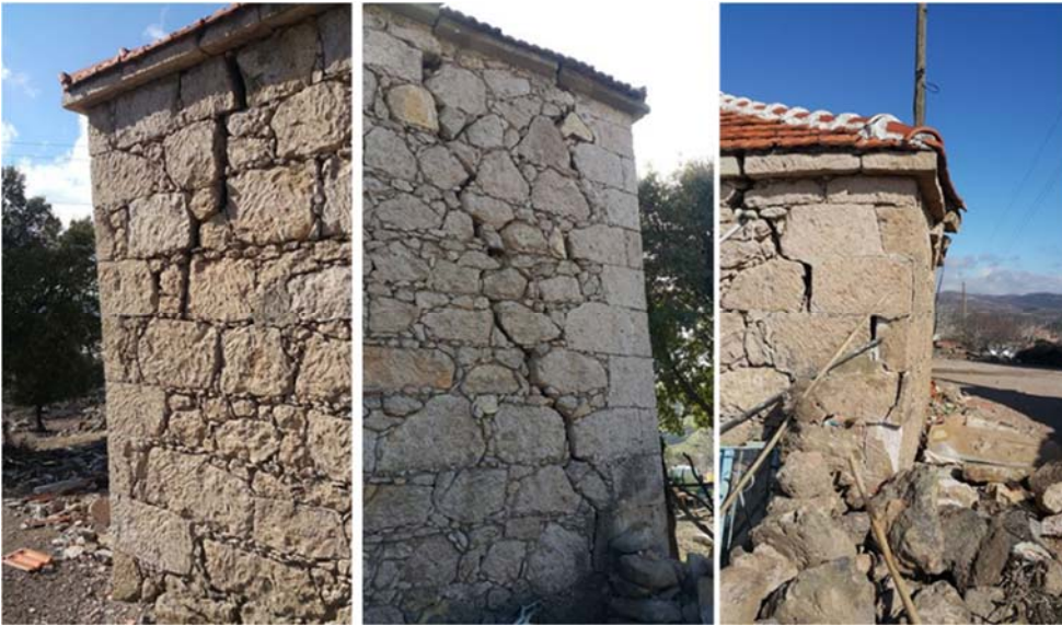
Figure 22 Examples of diagonal shear cracking
