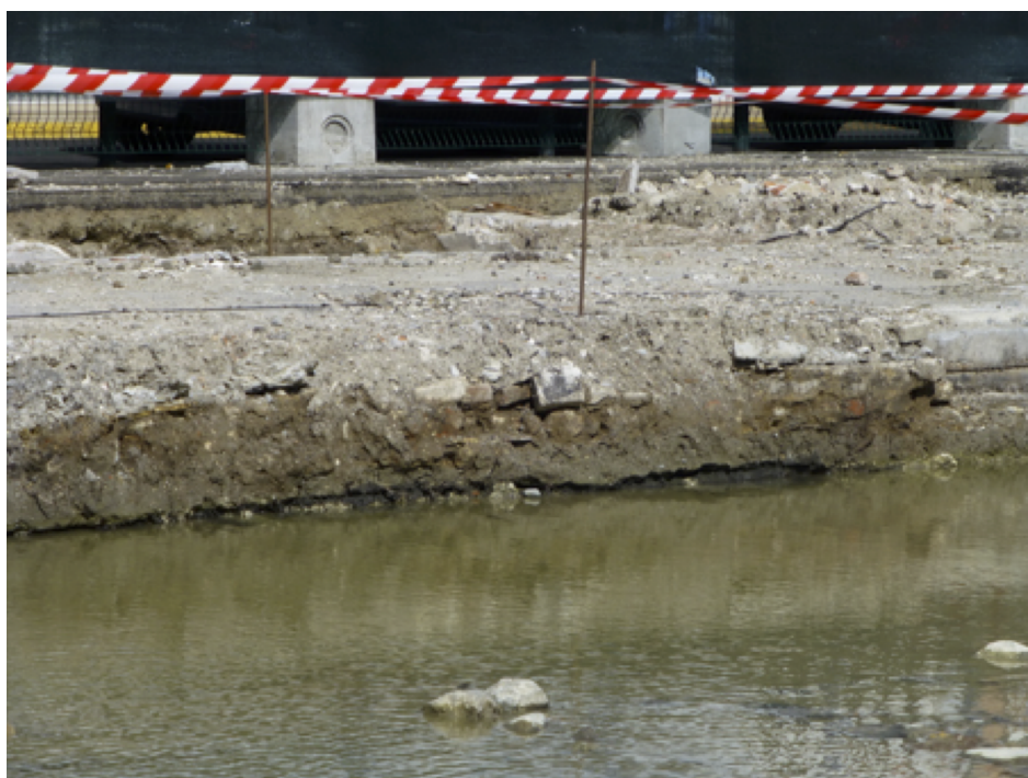
Fig. 5. The deposit layer is the dark layer just at water level
