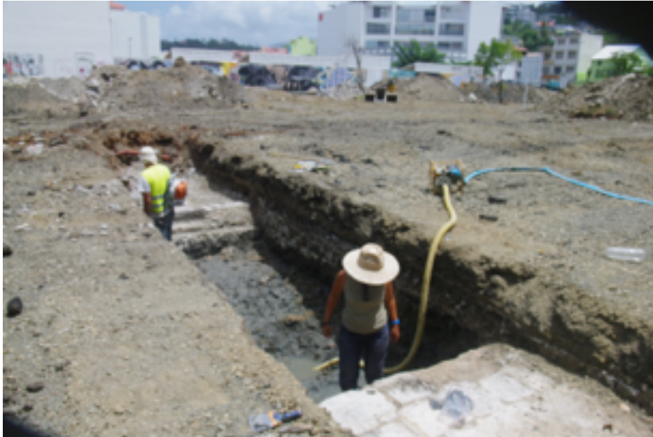
Fig. 6. The water pumps working at site 2, so that we could study the deposit.
