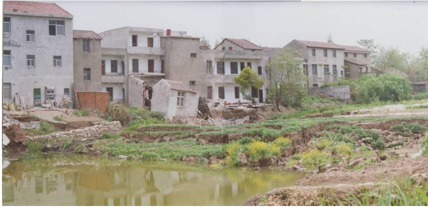
Fig.2. Damage scene caused by the cover-collapse sinkholes in Fenghuo Village in 2000
