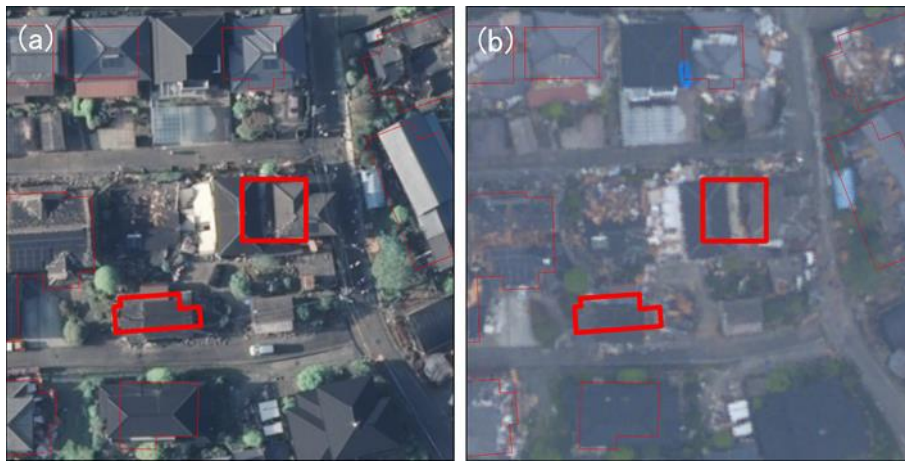
Figure 16: (a) Aerial image taken on April 15; (b) Aerial image taken on April 23. The thick red polygons shows buildings that collapsed after the foreshock and were detected using the \Delta H threshold.
