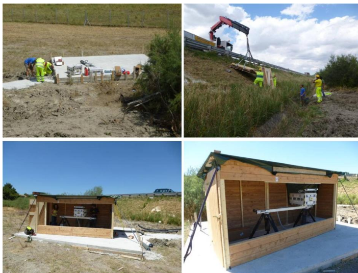
257 Figure 4. Pictures of the construction of the covered structure and installation of the GB-InSAR.
