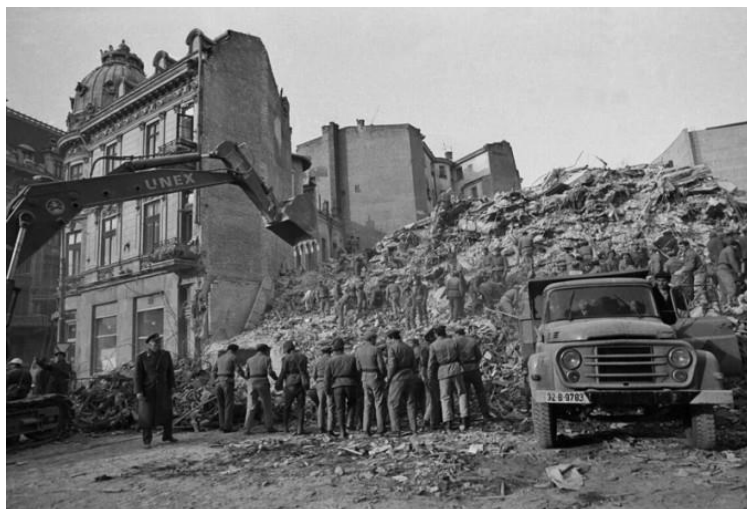
Figure 2. In 1972, the collapse of the Continental block in Bucharest's historical center blocked the access streets, so clearance was delayed by more than 12 hours; the photo shows efforts to identify survivors and property. Source: Agerpres.
