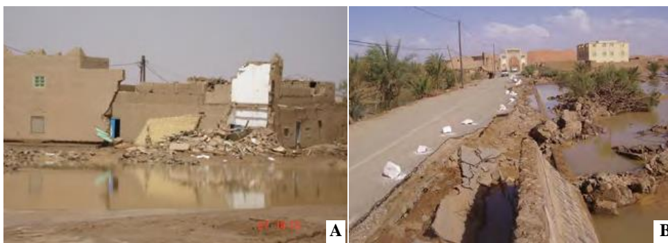
Figure 3: A: Collapsed houses in Merzouga. B: State of the road after a flood, at the entrance of Merzouga (Source: Kabiri, 2012).
