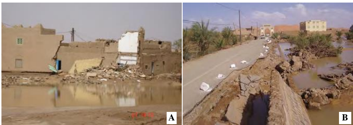
Figure 3: A: Collapsed houses in Merzouga. B: State of the road after a flood, at the entrance of Merzouga (Source: Kabiri, 2012).
