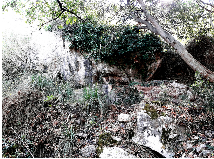
Fig. S3 – View of fallen rock blocks (Range of volumes: about 1.5 to 30 m 3 ) at the base of Lower Cliff.
