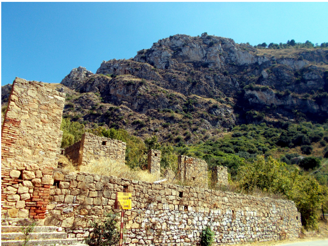
Fig. S2 – Ruins of the new thermal establishment of Sclafani (1856-57).
