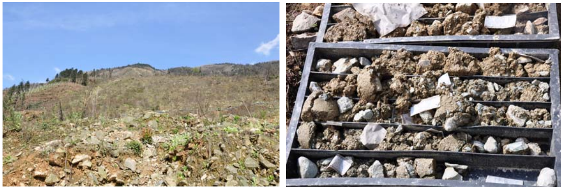
248 249 (a) Material on the landslide surface (b) Material in the shear zone
